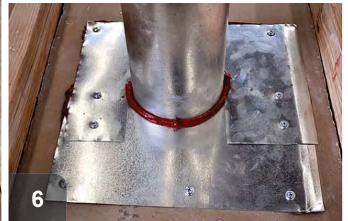
6 Fasten rigid material to cover penetration and seal against flue with caulk
