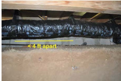
Flex ducts should have supports no less than every 4 feet
