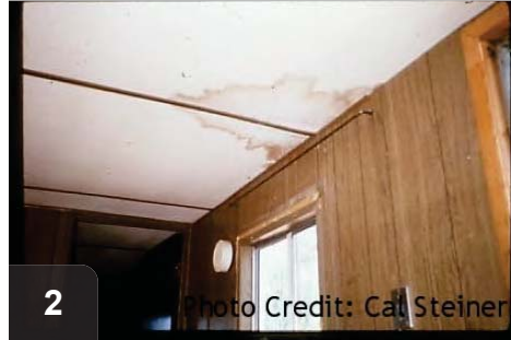
2 Inspect ceiling for weakness, leaks, clearance to combustibles, loose panels, and penetrations
