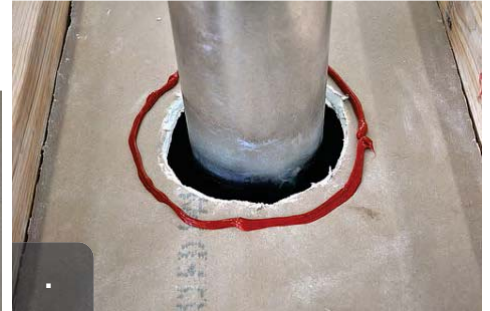
Apply first ring of caulking to match shape of opening
