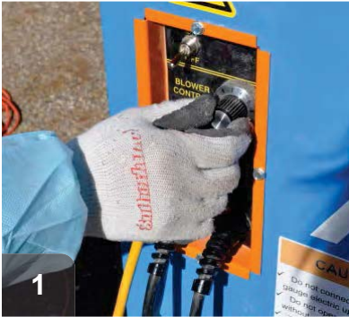
1 Adjust machine settings for loose fill: open gate for high material flow, allow enough air pressure to avoid clogging.
