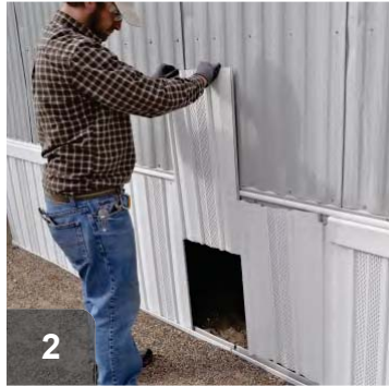
Reinstall skirting, if necessary
