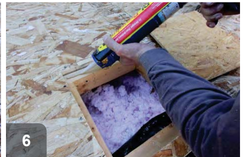
6 Apply subfloor adhesive to nailers
