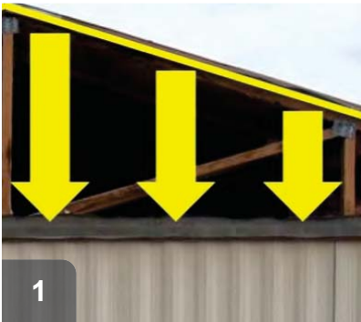
1 If insulation is roof mounted, blow below it.
