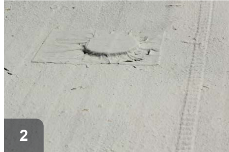
2 Inspect all patches and repairs, and correct deficiencies if necessary
