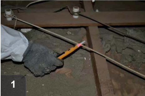
1 First determine whether K&T wiring is active using an AC voltage detector. The tip glows red for active wiring.
