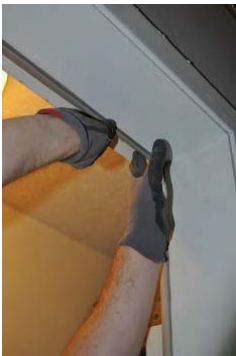
Corners of weatherstripping should be snug and secure
