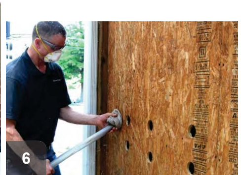
6 With a rag or fiberglass batt to prevent insulation blowing out, fill all cavities in exterior walls with insulation.
