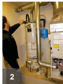
If spillage occurs, refer to Annex D on WA State combustion safety form.
