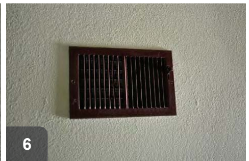
Once mastic is set, grill can be replaced and mastic should not show
