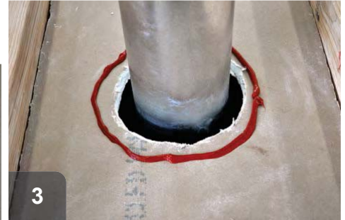
3 Apply first ring of caulking to match shape of opening
