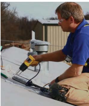
Use a heat gun to make the adhesive pliable to get the best possible seal.
