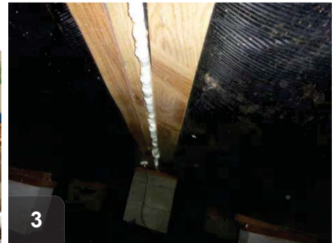
Foam sealant has been installed to air seal the floor plane marriage line, accessed from below.
