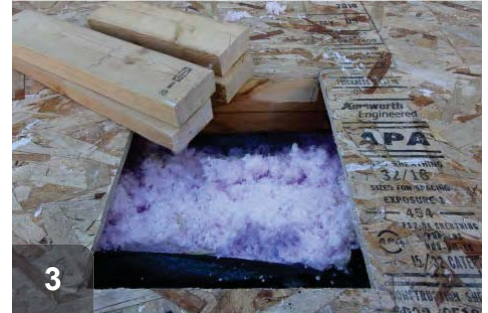
3 Cut four 2X4 blocks to support the patch
