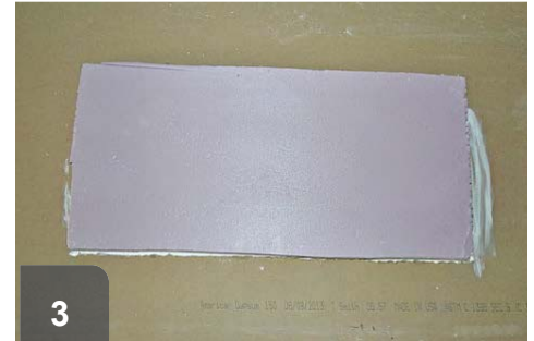
Trim rigid material, such as drywall or XPS, to size and place over sealant
