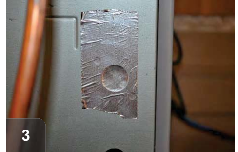
Fully cover holes with tape to seal completely
