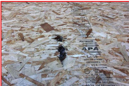
Remove floor coverings from damaged area
