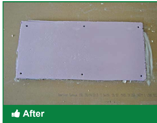
The air barrier is maintained by capping chases with rigid material
