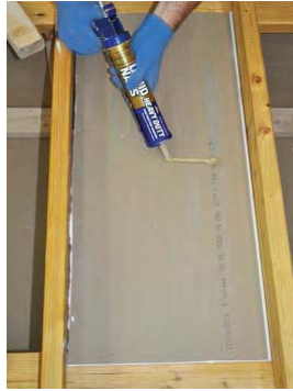
When supporting from above, apply adhesive between drywall and bracing
