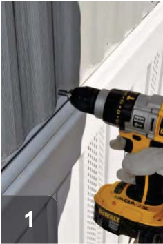
Using new fasteners, reattach paneling
