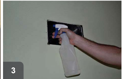
Wet the edges of the drywall to ensure a good bond
