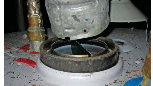
Inspect ventilation systems for disconnected pipes
