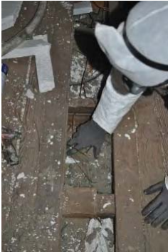
Check cavity for electrical junctions and penetrations
