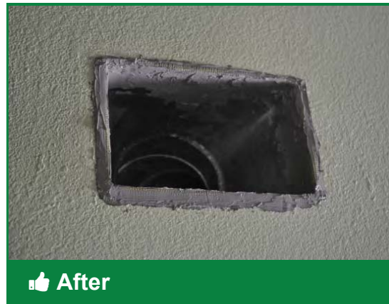
Use a mesh tape and mastic or UL 181 Aluminum Butyl Tape to seal duct boot to interior surface
