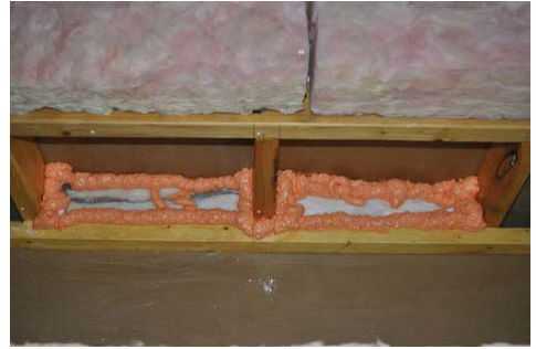
Option 2: Backing used to fill bays and sealed with spray foam
