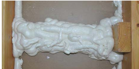
Option 2: Bridge cavities with spray foam
