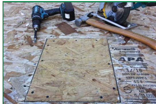
Completed floor repair
