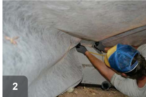
2 Secure netting across sills to prevent leakage of insulation
