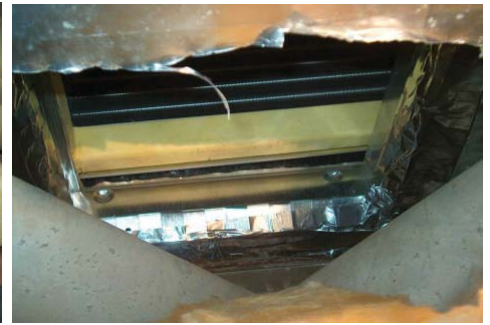
Create an opening large enough to completely seal the plenum to the trunk line.
