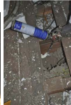
Seal any penetrations
