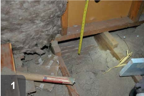
1 Measure floor joist opening so material can be cut and installed to prevent air leakage.
