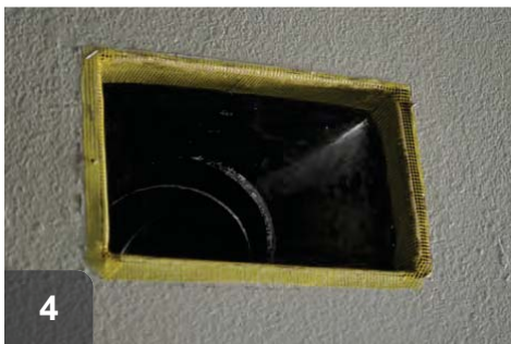
Cut mesh or UL 181 Aluminum Butyl tape to fit around duct boot and cover gaps
