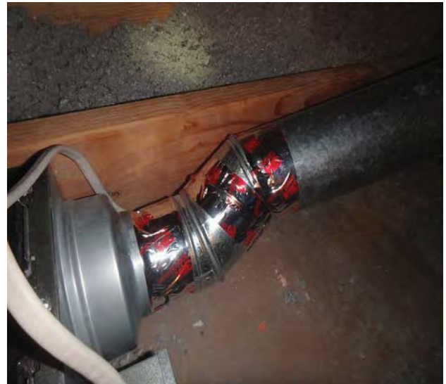
Seal exhaust fan duct seams with mastic of UL181 tape.
