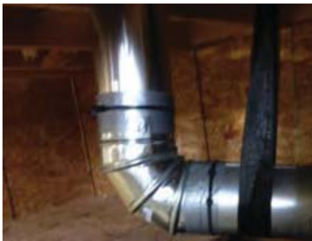
Rigid vent material supported with nylon strapping
