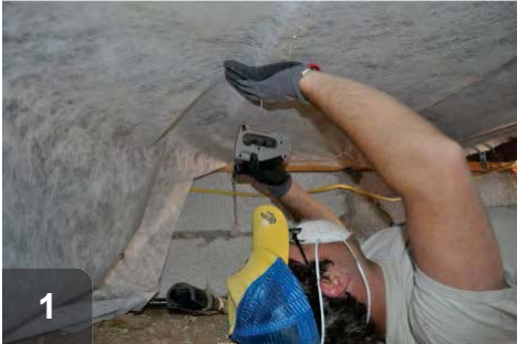
1 Secure netting across each joist to create separate cavities
