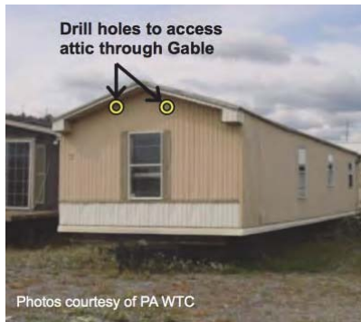
Locate the ceiling level and truss framing prior to drilling through gable siding.
