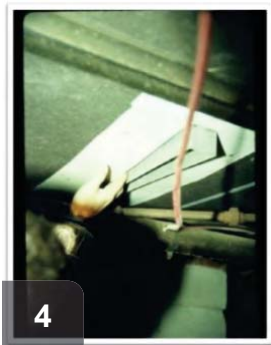
4 Maintain all combustion air intake openings when patching belly material.
