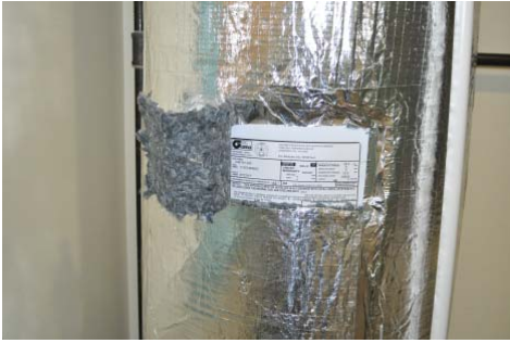
Data plate should still be accessible after wrapping
