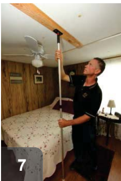
7 Use temporary supports to avoid ceiling collapse during insulation install
