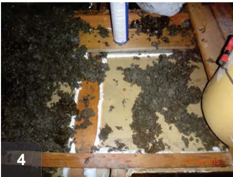
4 Top plate sealed to ceiling material.
