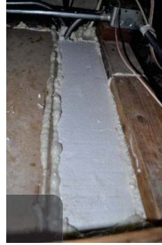
Sealant is used to fill in all cracks and gaps along edges of chase cap. Cap is now sealed.
