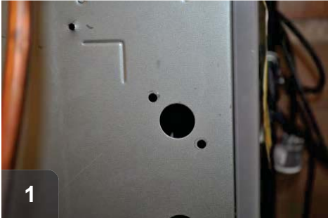
Unnecessary holes in the air handler cabinet should be sealed
