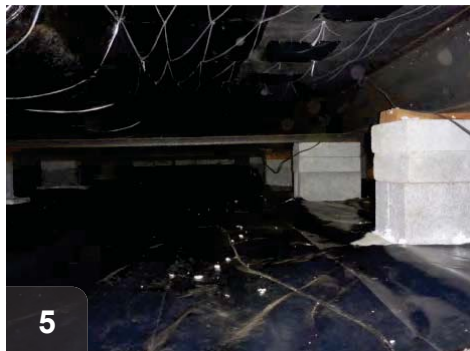
5 Pin up sagging belly material to prevent installing excessive amounts of insulation material.
