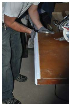
Ensure door sweep fits tightly against bottom of door and fasten in place
