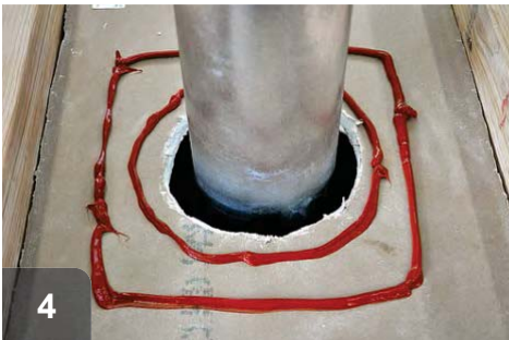
4 Apply second ring of caulking to size and shape of rigid material
