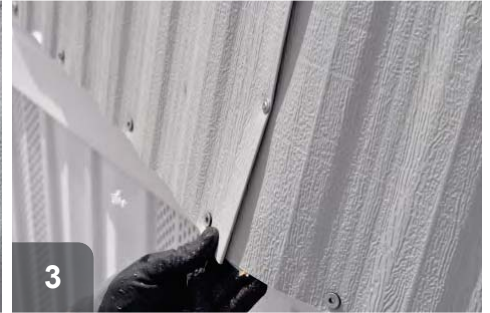
3 Seam should remain together with temporary fastener
