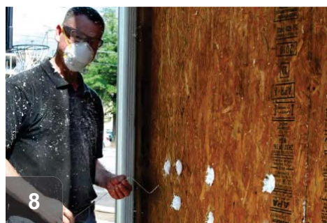
8 Check that cavities are filled and are the proper density.
