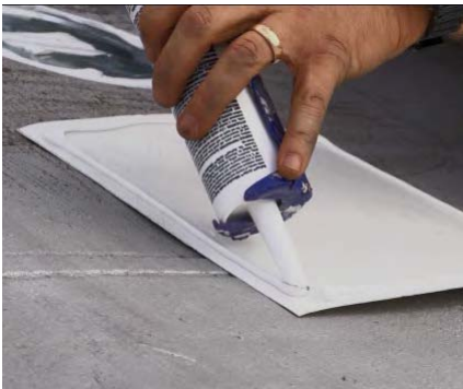
Apply sealant to the underside of the sheet metal patch.
