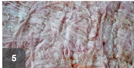
Insulate over now-capped soffit
