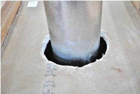
Gaps around flues and penetrations need to be sealed before insulating
