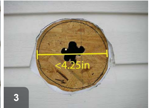
3 Clear wall surface and mark hole size 1/4" larger than termination fitting
