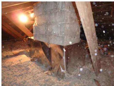
Damming is held in place with mechanical fasteners and maintains 3" clearance from chimney.
