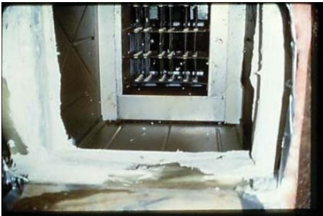
Using mastic and mesh tape, fully seal the furnace to the trunk line. Patch opening in duct with sheet metal and seal. Repair and seal the access holes in duct and belly.
