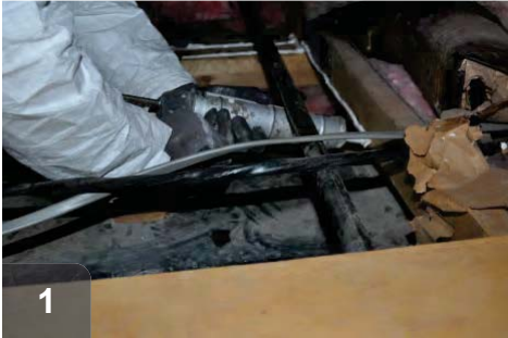
1 Apply sealant to surrounding surfaces before setting cap in place
