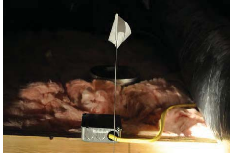
Flag and install covers on electrical junctions
