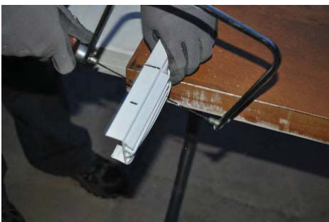
Cut door sweep to width of the door
