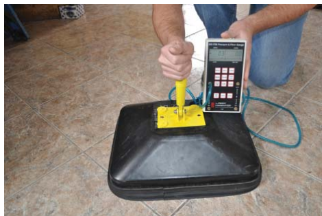
As with all duct sealing and repair, confirm success with pressure diagnostics.
