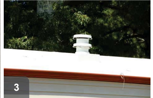
3 Verify presence of rain caps on all vents
