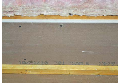
Soffit now properly sealed from attic with drywall, sealant and fasteners
