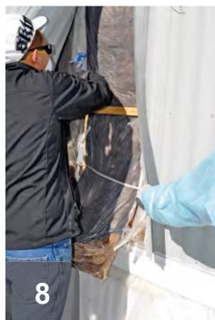
8 Tuck bottom of batt behind bottom belt rail. If longer than cavity, cut to within 1" longer, roll and tuck into cavity
