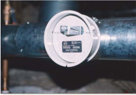
Determine if a draft regulator is installed and working
