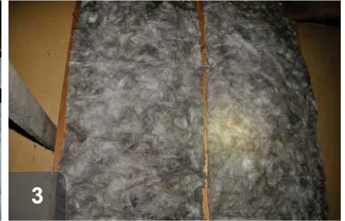
3 Batts should fill entire volume of knee wall stud bays
