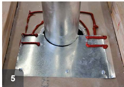
5 Fasten rigid, non-combustible material and apply additional caulking
