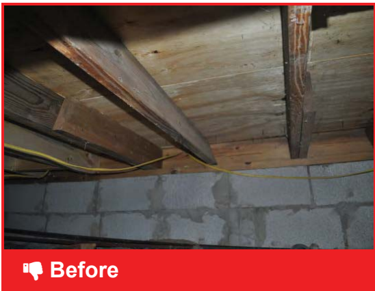
Before Uninsulated floors above unconditioned spaces are an energy drain
