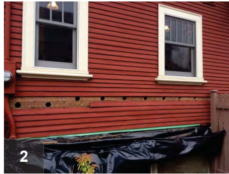
2 Remove siding and drill holes in sheathing for installing insulation. Follow lead safe work practices when needed.
