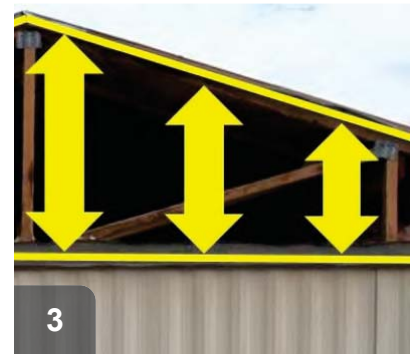
3 If insulation is mounted at both the ceiling and the roof, blow between it.
