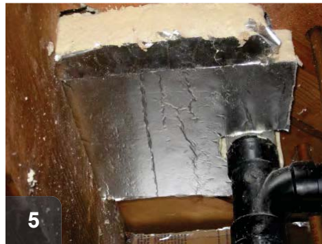
Seal large tub chase using rigid, sheet material (foam board, sheet metal, plywood, etc) then caulk or foam edges
