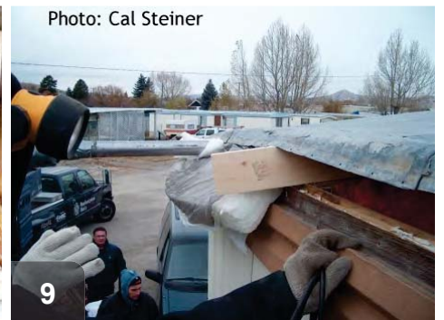
9 After opening the roof edge, verify proper clearance to combustibles and inspect vent connections
