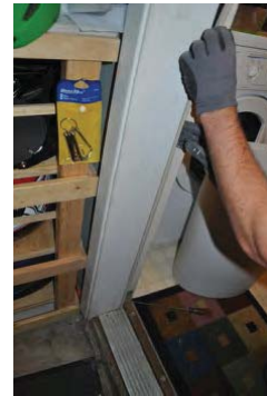
Install weatherstripping into rabbit around door
