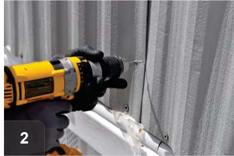
2 Temporarily fasten siding panels at joint to hold seam together
