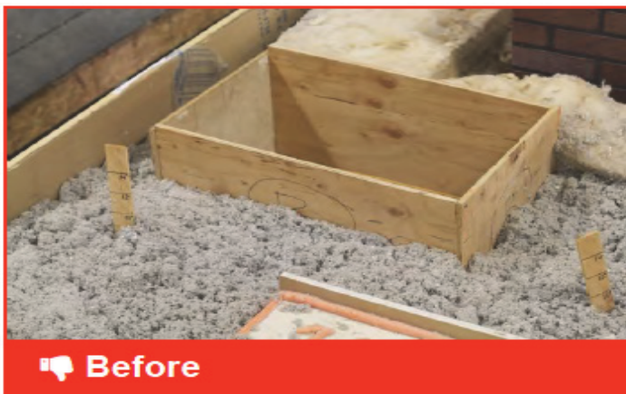
Uninsulated attic hatch
