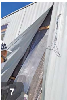
7 Beginning with lapped end, tuck batt under top belt rail and stuff batt up to top of cavity. Remove stuffing tool
