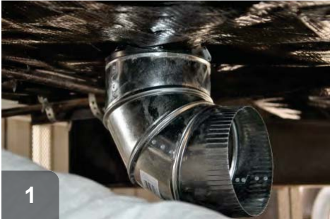
1 Attach elbow duct and orient in correct direction to minimize duct run
