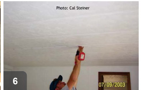
6 Repair and refasten sagging or unsecured ceiling panels. Caulk and seal seams to prevent insulation spilling into house
