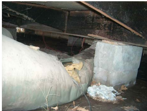
Removing the crossover duct may provide access to the plenum. Replace and seal the crossover duct after sealing plenum
