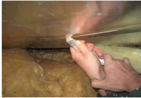
Cut belly to expose duct trunk. Use a utility knife to cut access under furnace plenum
