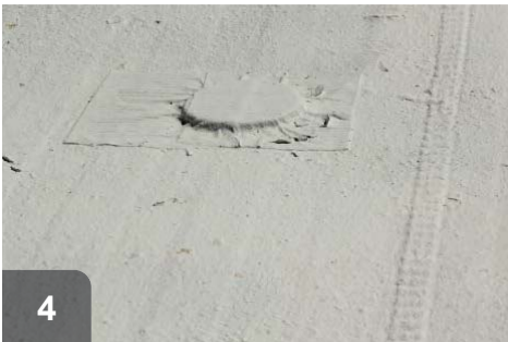
4 Inspect all patches and repairs, and correct deficiencies if necessary
