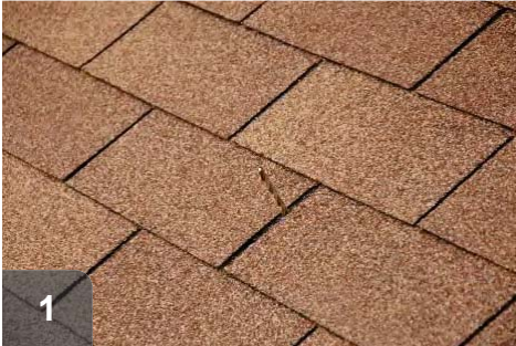
1 Locate the center of your vent hole by drilling from inside through roof
