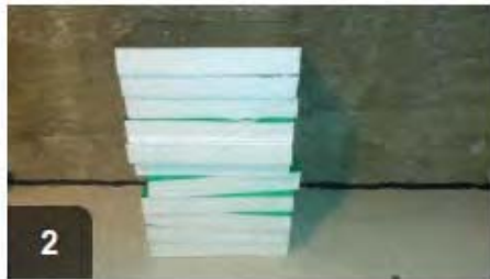
2 Save time by pre-cutting pieces of rigid foam to fit between floor joists. Gaps will be air sealed.
