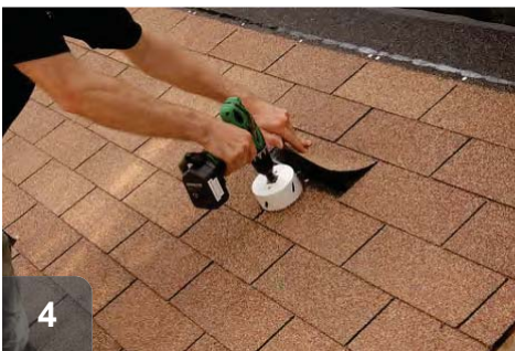
4 Hole should be no more than 1/4" larger than termination fitting diameter
