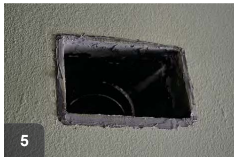
Apply mastic over tape to create heat resistant, durable bond
