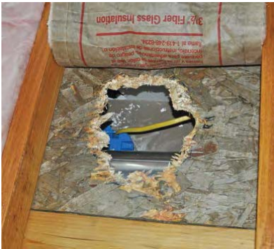
Prepare work area by removing existing insulation and debris
