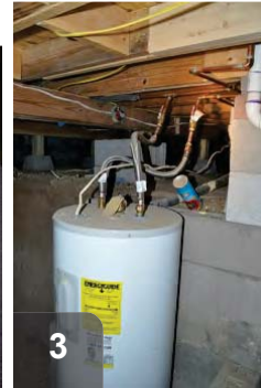
3 Adjust water heater settings and insulate as needed
