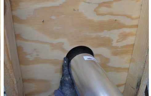
Collared fittings extend through the roof to fasten securely with duct
