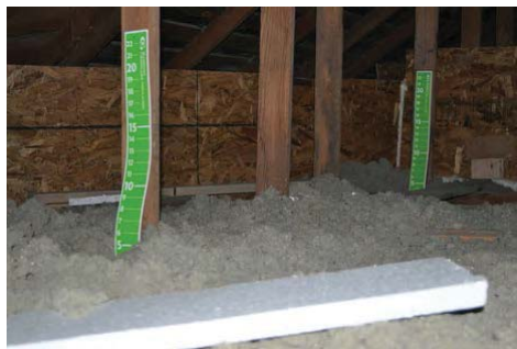
Install depth markers and insulation dams above height of insulation
