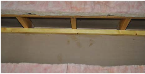
Clear work area of insulation and debris
