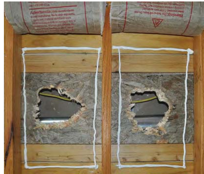
Option 1, Step 1: Run a bead of sealant around damage in old ceiling
