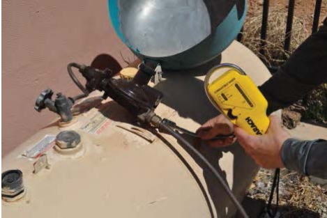
Check all raw fuel lines for leaks
