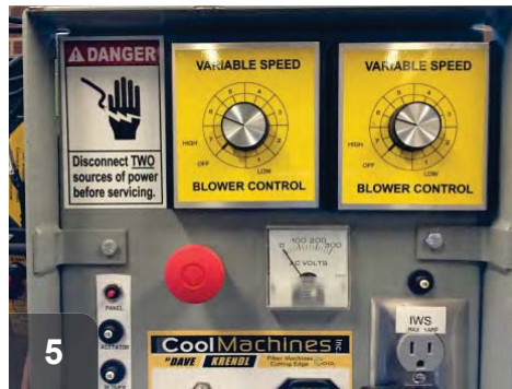
5 Adjust the pressure (controls shown here) and the feed gate to fill an 8-foot wall cavity in 2 to 4 minutes.
