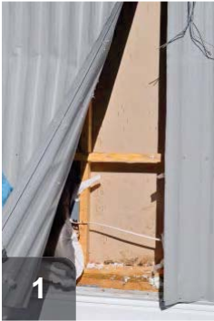
1 Uninsulated wall cavity can be accessed from exterior of mobile home through paneling
