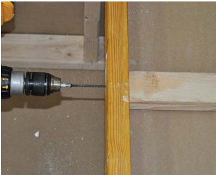
Ensure new bracing is secure by using screws to fasten to joist
