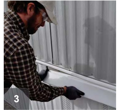
Reattach trim, if necessary
