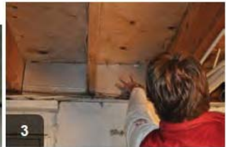
3 Pressure fit rigid insulation into
