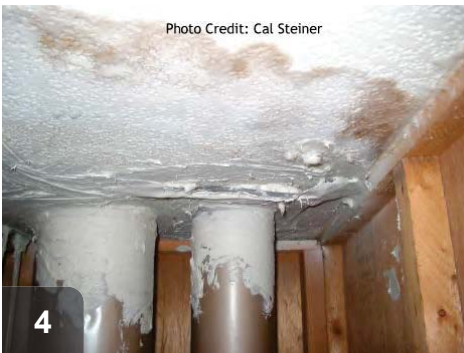
4 Inspect ceiling for weakness, leaks, clearance to combustibles, loose panels, and penetrations
