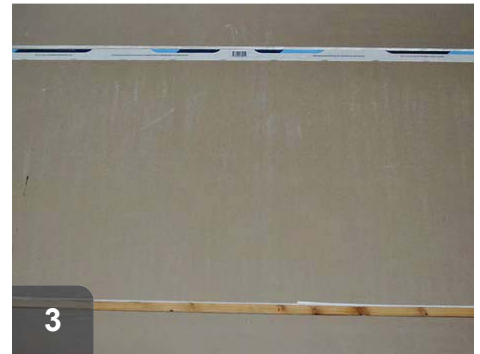
Cap soffit with rigid material, such as drywall, cut to size
