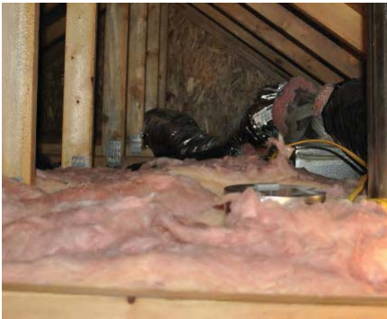
Perform visual inspection of confined spaces before beginning work
