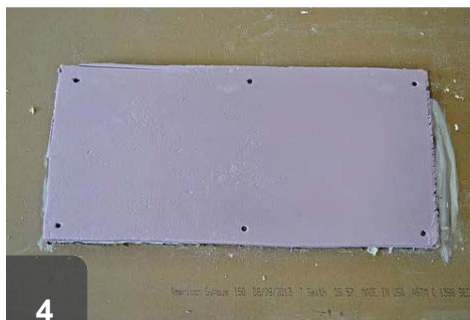
Fasten rigid material appropriately, such as with screws
