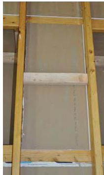
Once chase is capped, it is now ready to be sealed along framing
