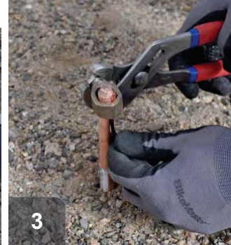
3 Attach grounding wire to rod with coupler
