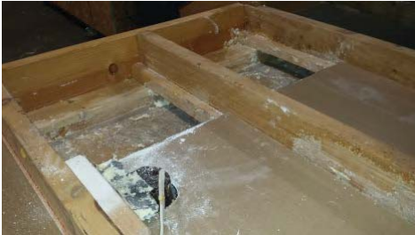
Soffit open to attic
