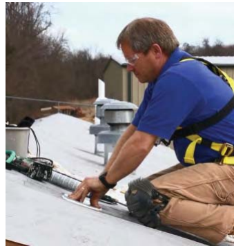
Firmly push the plug into place, until it is flush with the roof surface.
