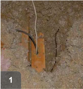
1 Locate wall tops in attic and look for plumbing and electrical penetrations.
