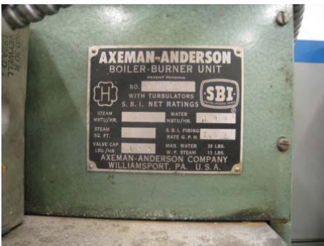
Check occupant's water heater model to see what r-value is built-in
