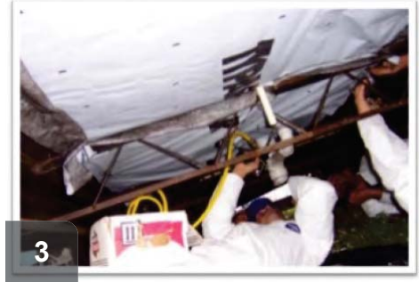
3 Workers install new material where rodent barrier is missing.
