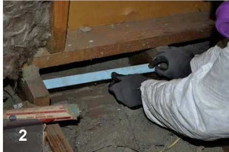
2 Install blocking to prevent air leakage.
