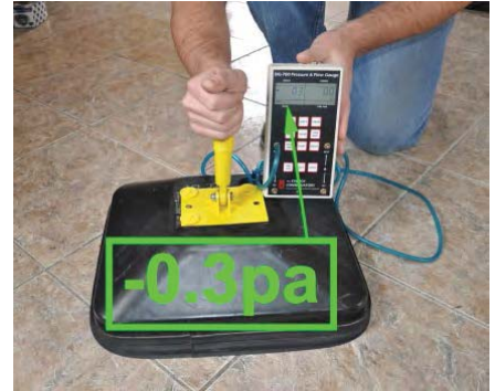
Perform pressure pan test after work is completed and compare to 'before' reading
