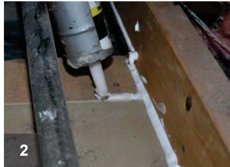
2 Sealant should extend along adjacent framing and into seams at top plates
