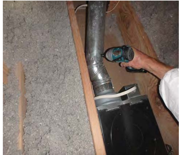
Fasten fan ducting with minimum of three screws at each connection.
