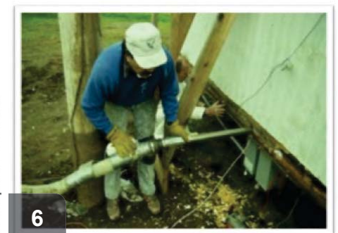
6 Belly cavity blown by drilling through rim joists.
