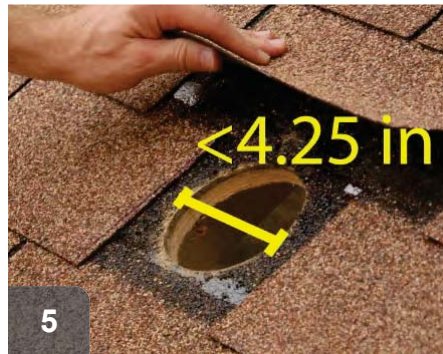
5 Verify hole size is correct before installation
