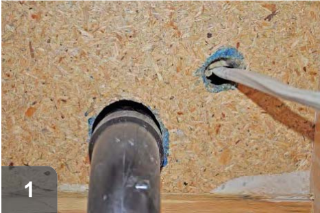
Locate gaps around penetrations for plumbing, electrical, etc.
