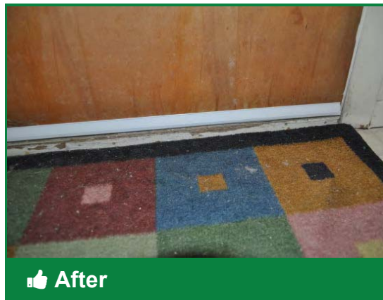
Door sweep, with weatherstripping, will minimize air exchange with garage
