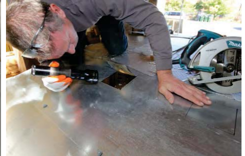
Regardless of access method, visually inspect attic for existing insulation, wiring, flues, obstructions, and hazards
