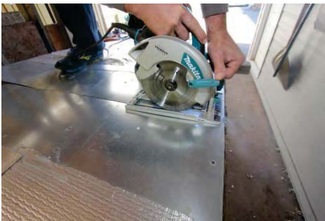
Another option: cut the roof open along the highest point from end to end. Make crosswise cuts at each end if needed
