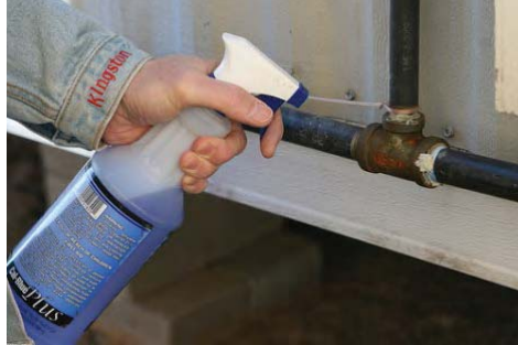
Use multiple methods to test for leakage--bubble solution
