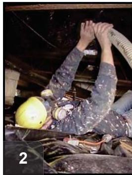
2 Loose fill insulation is blown into mobile home belly cavity.
