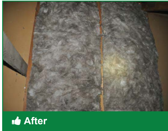
After Properly fit insulation filling full volume of stud bay
