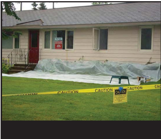
Exterior lead containment elements
