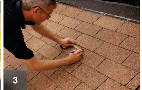
3 Based on termination fitting size (in this case, 4"), mark to cut hole
