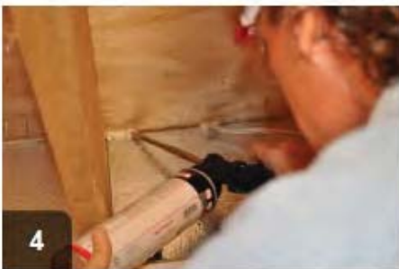
4 Air seal all seams where insulation meets framing.
