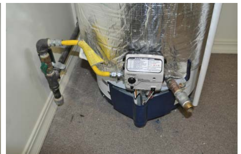
Wrap does not obstruct ventilation, thermostat access plate, hi-limit switch, or fuel line
