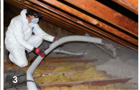
3 PPE for attic includes N-95 respirator or greater, gloves, and coveralls.
