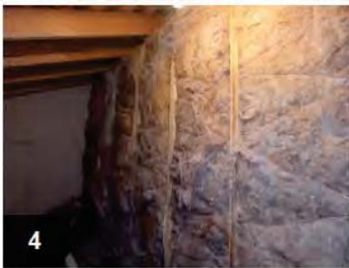
4 Knee wall insulation is supported by nylon, stapled in a zig zag pattern, 12" on center.
