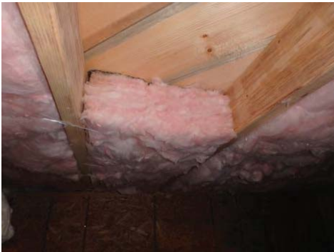
Batt must be in contact with subfloor without being overly compressed.
