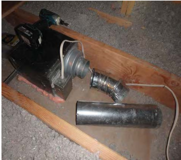
Assemble fan ducting.
