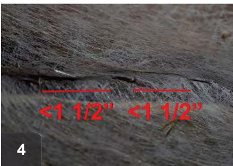
4 Staples should be kept tightly together, placed no more than 1 1/2" apart
