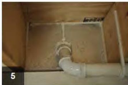
5 Cut insulation to fit around utility penetrations in rim joists. Air seal all seams.
