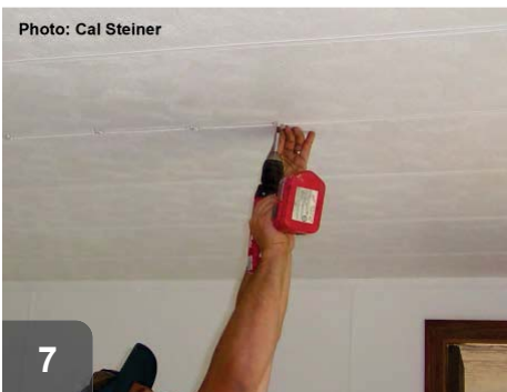
7 Add fasteners wherever needed to firmly attach ceiling to the trusses
