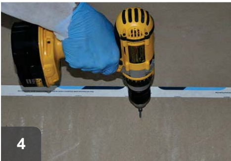
Fasten cap with screws to set sealant and create air barrier
