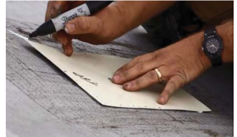
Use a 10"x10" sheet metal patch to mark the center of the hole.
