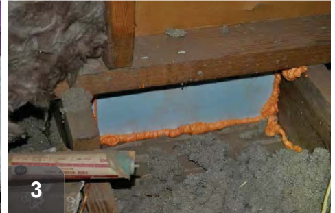
3 Blocking material is sealed to surrounding joist and framing
