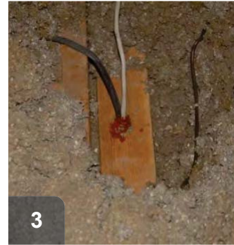
3 Sealed wall top penetration.
