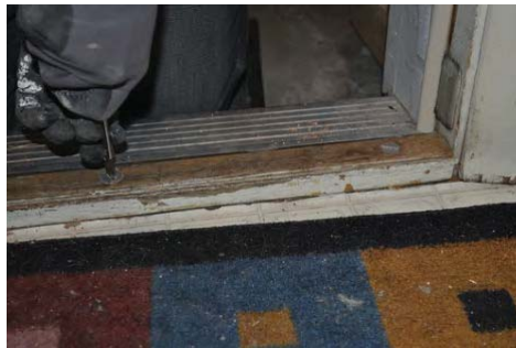
Adjust threshold to minimize contaminant and water infiltration
