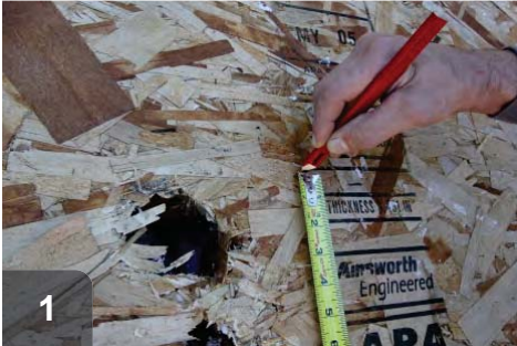
1 Mark the joist locations on either side of the damaged area
