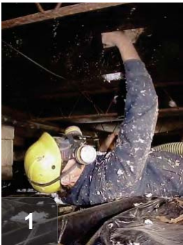
1 Holes are cut through rodent barrier (belly material) to insert insulation blow hose.
