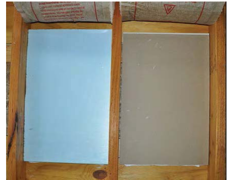
Option 1, Step 2: Cover openings with rigid material, either XPS or drywall
