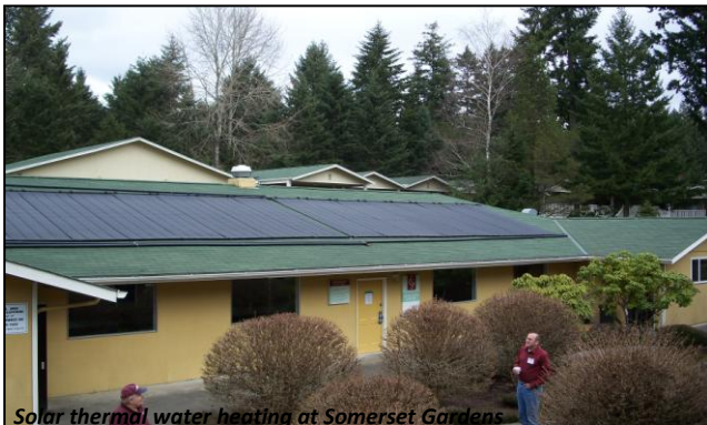
Solar thermal water heating at Somerset Gardens
