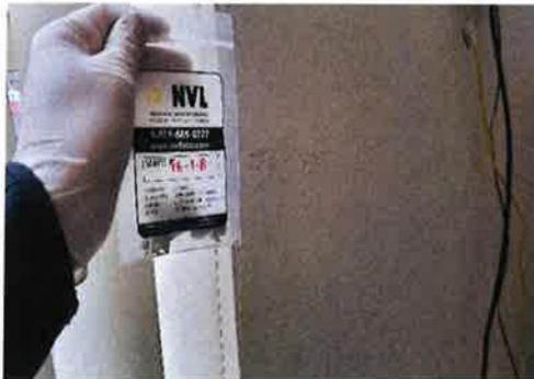
There is approximately 1200 linear feet of asbestos-containing joint compound with paint associated with the interior GWB walls that would be impacted during the renovation.
