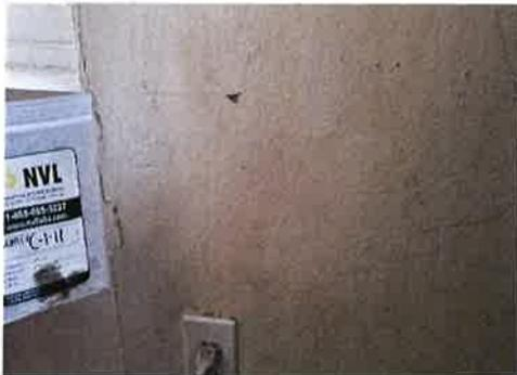
There is approximately 800 linear feet of asbestos-containing joint compound with paint associated with the interior GWB walls that would be impacted during the renovation.
