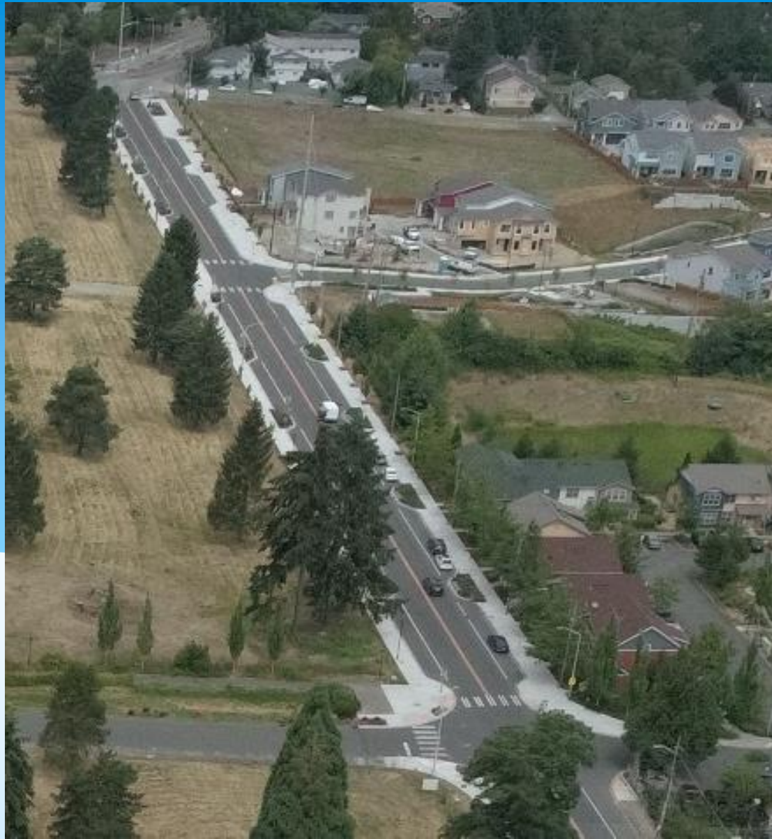
Completed 4 th Avenue SW Improvements Looking North
