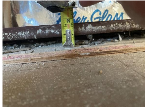
Photo 2. Metal Stud Wall separated from the concrete slab on grade approximately \frac{3}{4} ".
