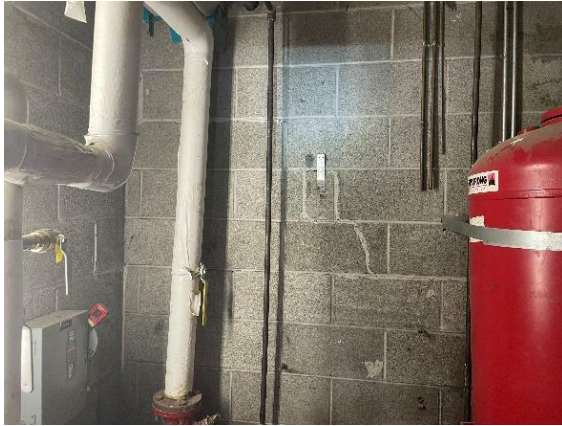
Photo 1. Typical cracks at masonry wall – Mechanical Room
