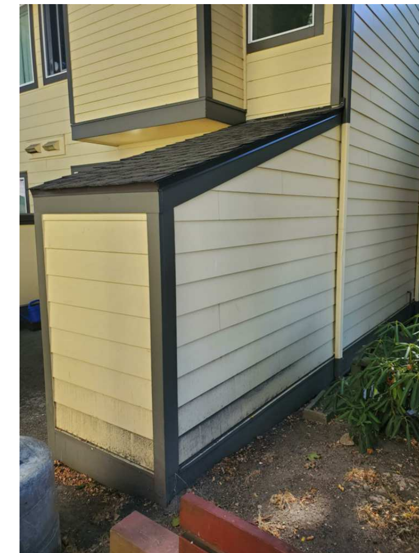
6 SHED EXTERIOR CORNER PHOTO NTS
