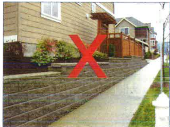
This inappropriate wall lacks base planting or interesting detail.
