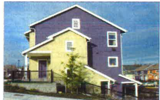
This building provides good grade transition by placing units on the upper and lower grades.
