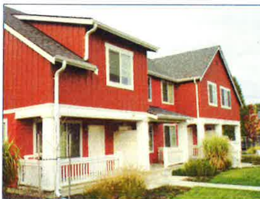
A good example of clear entries and deep porches.
