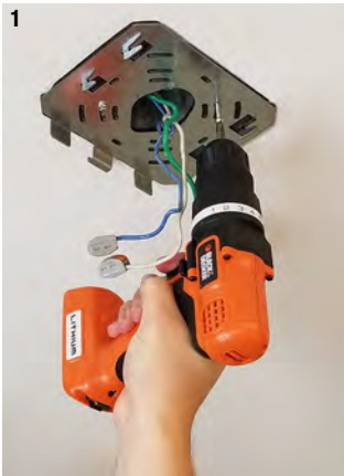
1 Mount plate to junction box.
