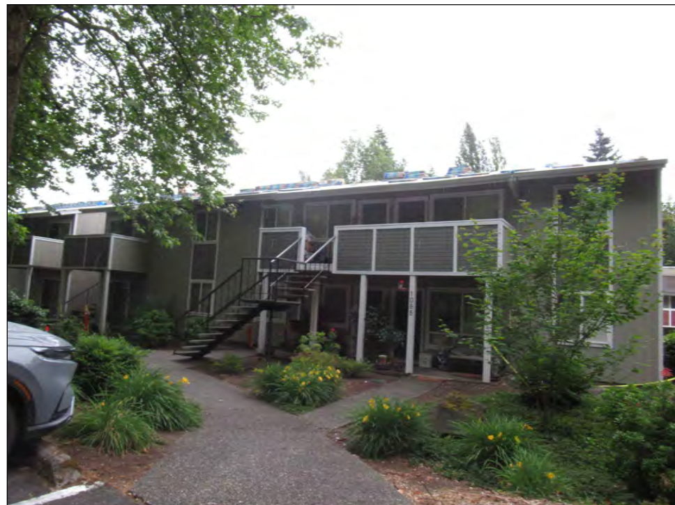
FRONT ELEVATION OF BUILDING
