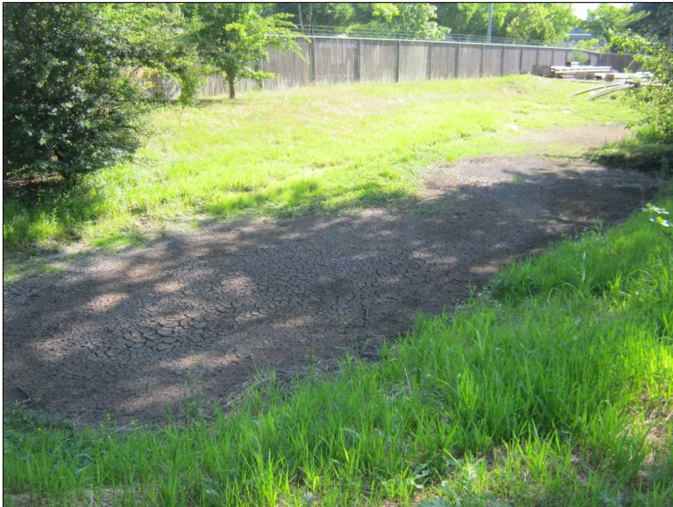
17. Artificial stormwater retention pond
