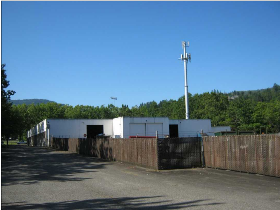
1. Subject Property viewed from the northeast
