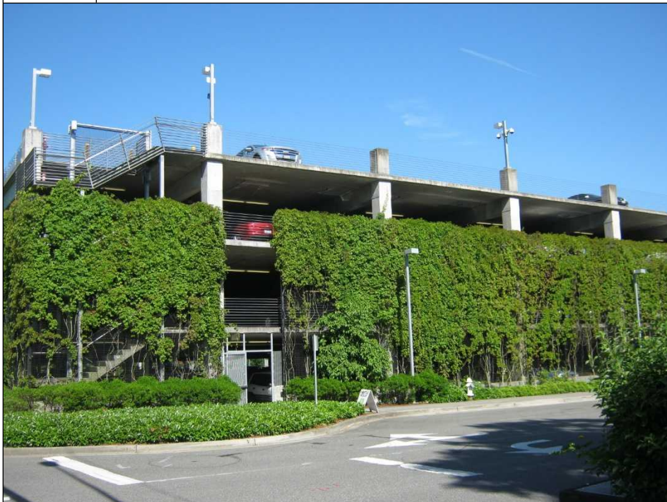
24. Adjacent parking structure to the west
