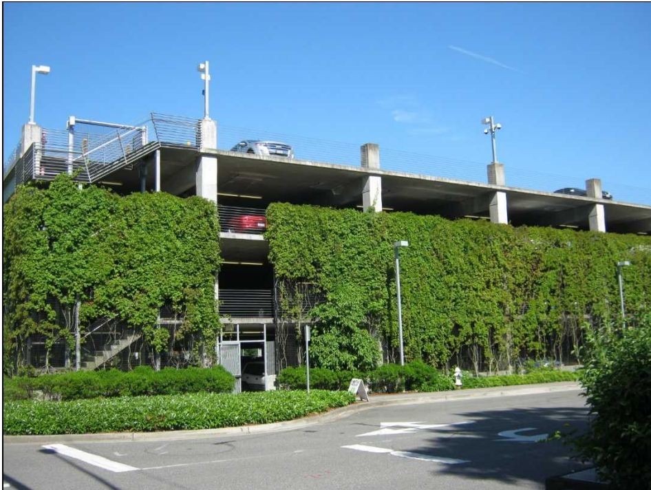
11. Adjacent parking structure to the west
