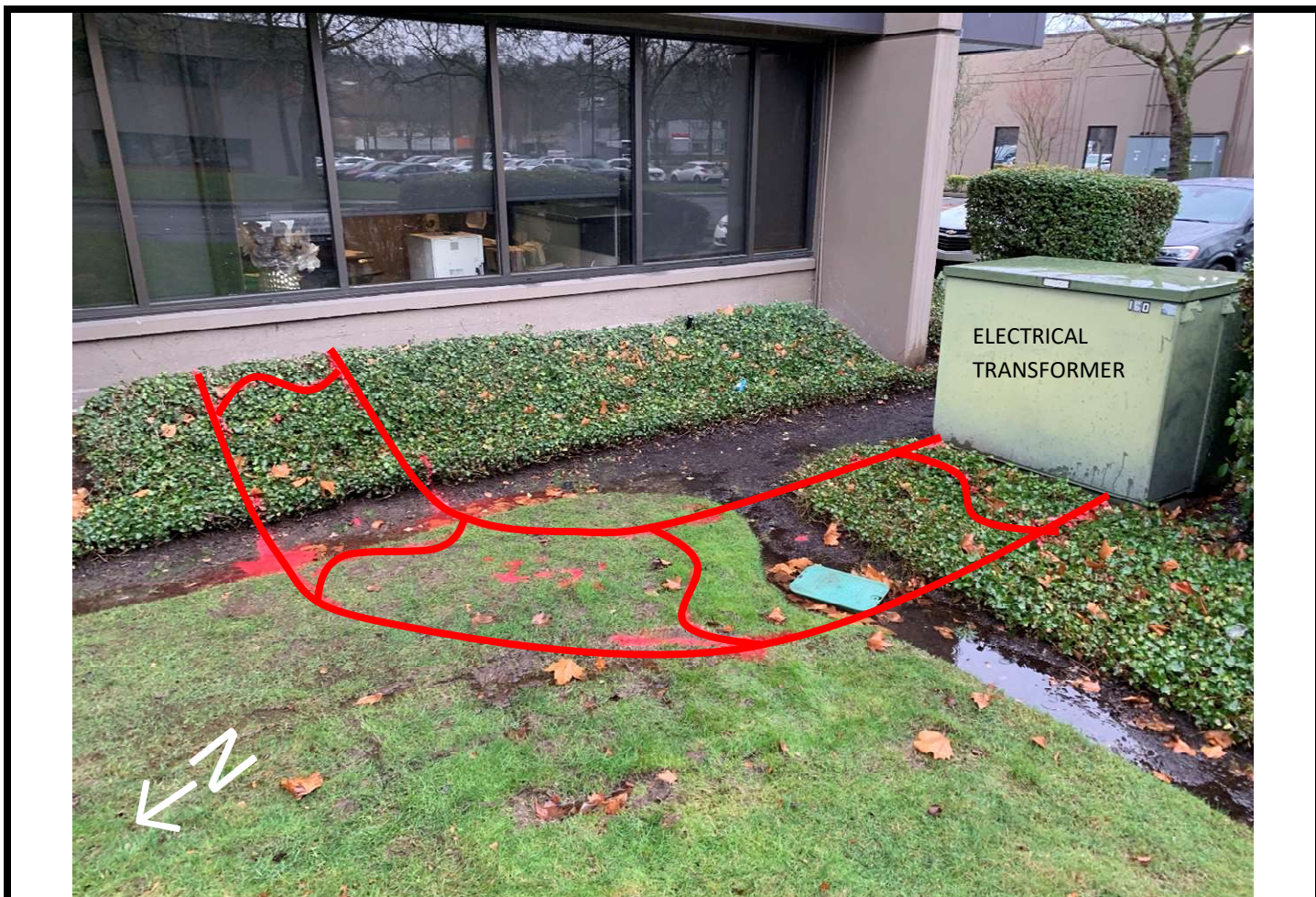
Photo taken in site showing rear of transformer and electrical duct. This electrical duct was identified as being the same one located in the lobby. In this area, lines are between 1'-2' deep.
