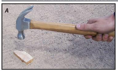
**A.** Using a string line, drive 3 inch stakes along the path of the drain every 30 inches.
