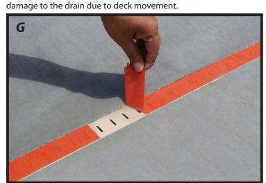
**G.** Remove the protective tape after the concrete installation is complete.
