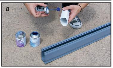
**B.** Using P.V.C. primer and cement on both the drain and the couplings, weld them into one piece.
