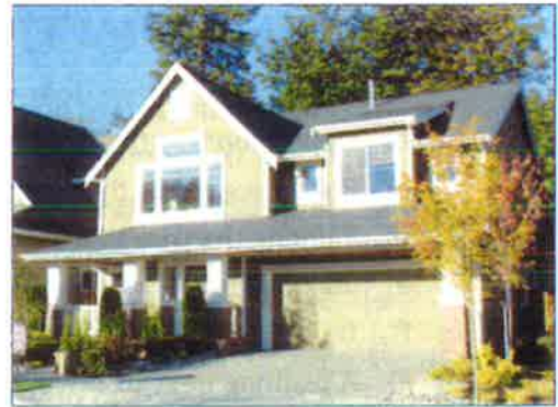
The presence of this 2-car garage is reduced by putting it on the same front plane as the rest of the house and the significant eave, which unifies the whole house architecturally.
