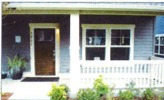
Cost effective use of trim in detailing at home front, where it will be regularly seen and appreciated. Note porch light, door, post band, and lintels.
