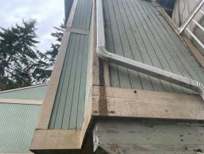
Pictures below are examples of areas on the building showing significant wood deterioration/rot or damaged on siding, trim and railings. These issues should be addressed during the preparations to be repaired/replaced, prime and paint according to specification.
