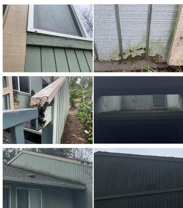
Pictures below are examples of areas on the building's underside plywood showing mildew/algae, mold, debris, damages, disrepair and spray paint tagging. These issues should be addressed during the preparations to be repaired/replaced, prime and paint according to specification.
