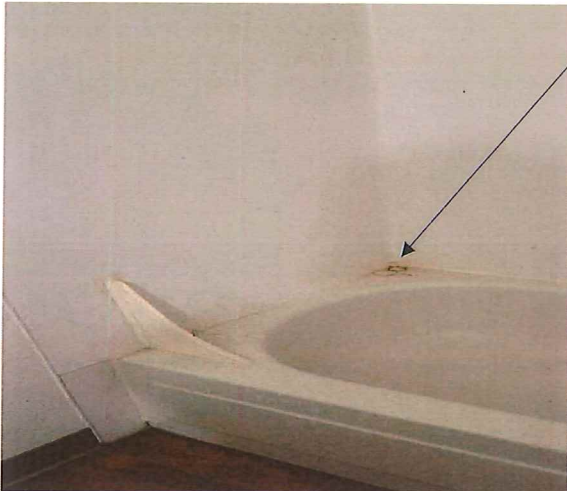
The white caulking in the restroom tested negative for asbestos. The caulking was also observed on the quartz countertop.
