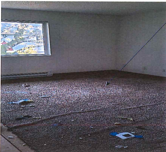
The carpet mastic inside of the bedroom tested negative for asbestos.
