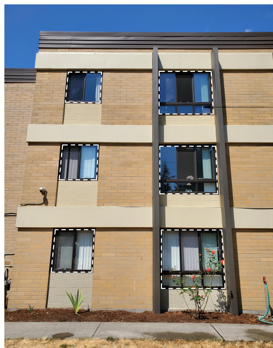
PHOTO @ PORTION OF NORTH ELEVATION
