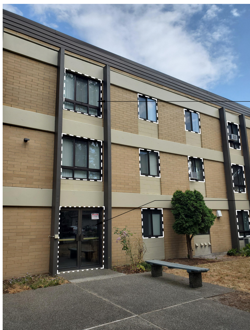
PHOTO @ PORTION OF WEST ELEVATION
